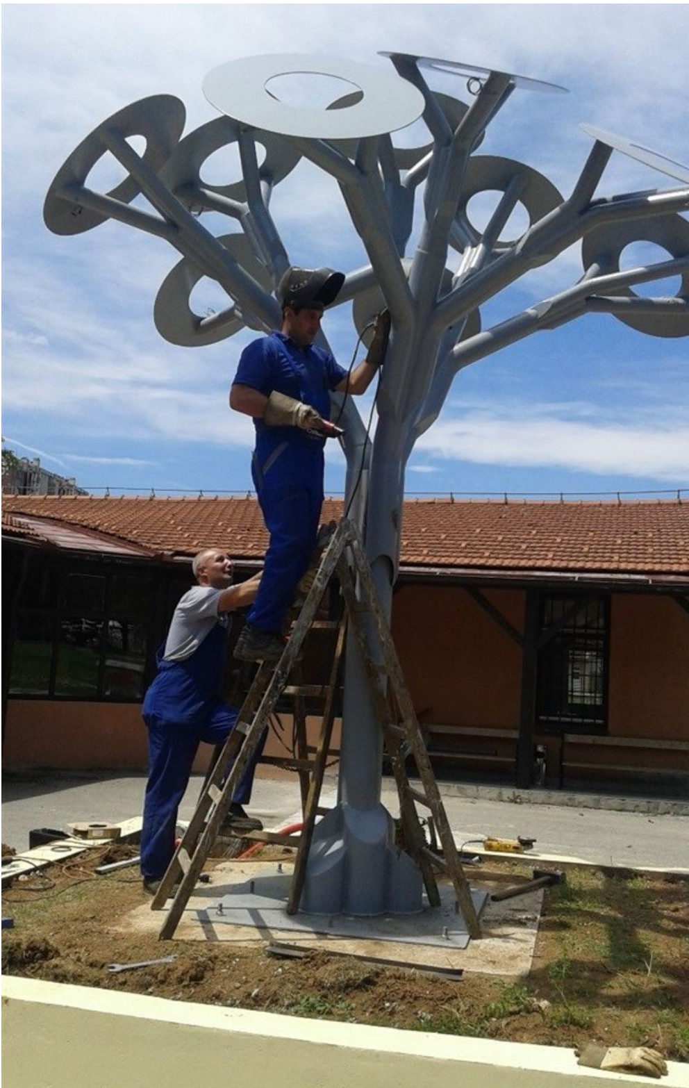
Installation of a solar tree on Sarajevo University campus. Image source: IEEE Project
