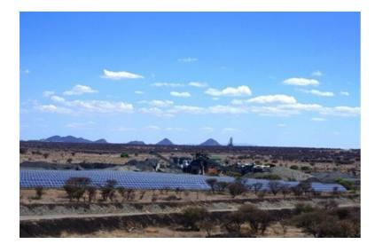
In these power plants diesel consumption is reduced through the integration of a photovoltaic power plant. In comparison to traditional grid-connected PV power plants the engineering requirements are much higher.
