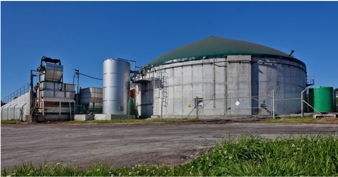
The digester at Elgin Fruit Processors that converts fruit and other waste to electricity. (Image Supplied)
