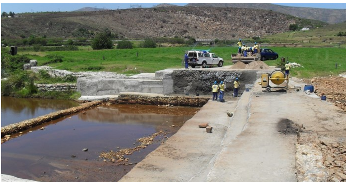
Image Supplied: Teams employed by Gamtoos Irrigation Board construct concrete weirs and other structures to conserve degraded peat wetlands in the Kromme River system.
