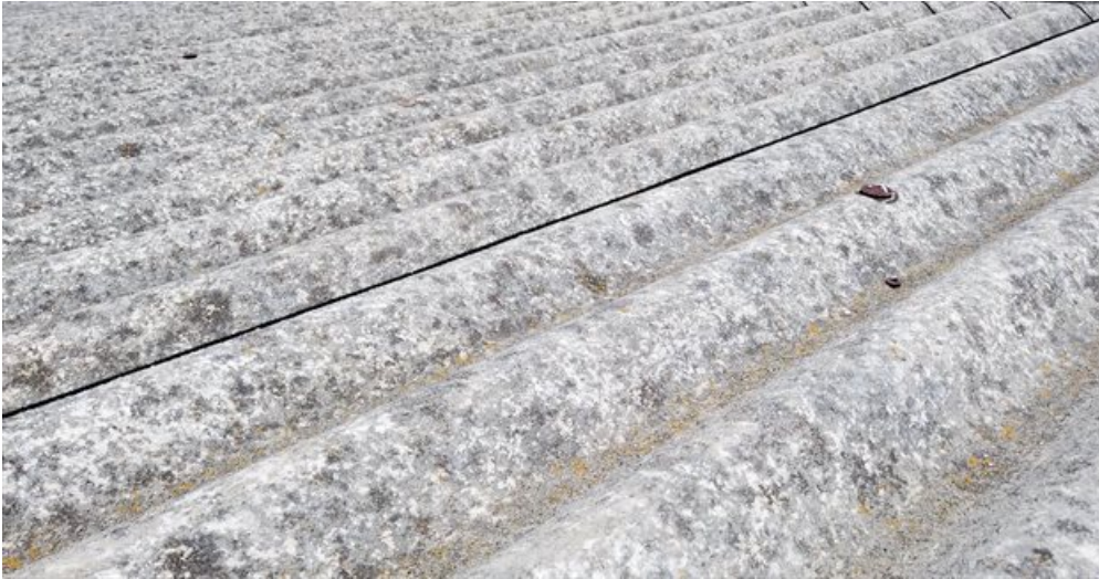
Asbestos roof sheeting. Image supplied
