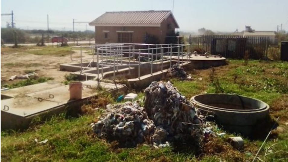
Objects flushed into the sewers that clog the system stand in heaps at the pump station in Valencia, Addo. | Photo: Joseph Chirume
